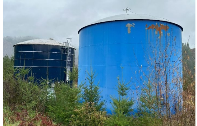
FIGURE 3-3: EXISTING WATER STORAGE TANKS
